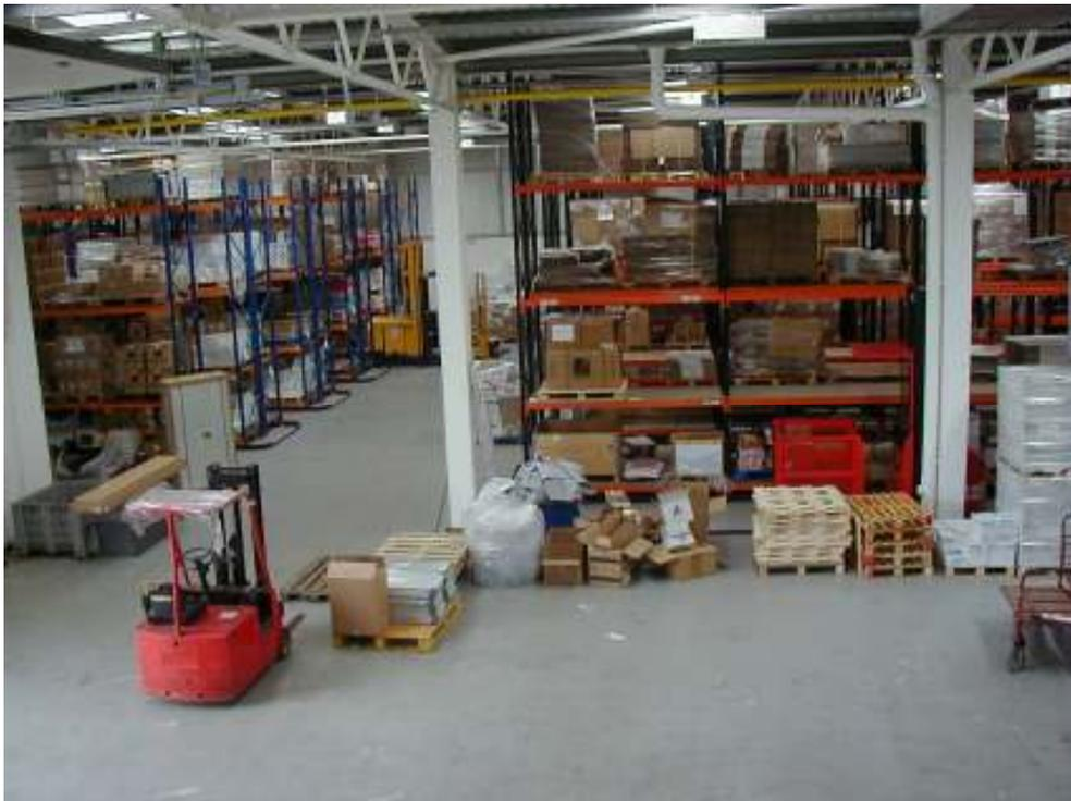
Due to the poor state of the existing polyurethane coating, Ryebrook spent considerable time shot-blasted the floor in three sections before diamond grinding to a smooth finish. All holes were then made good using Ryebrook's mortars and fillers. Having prepared a suitable surface, the Ryetech coating was laid to a 0.5mm thickness in the warehouse, with Ryeflow being laid to all other area at a nominal 2mm.
